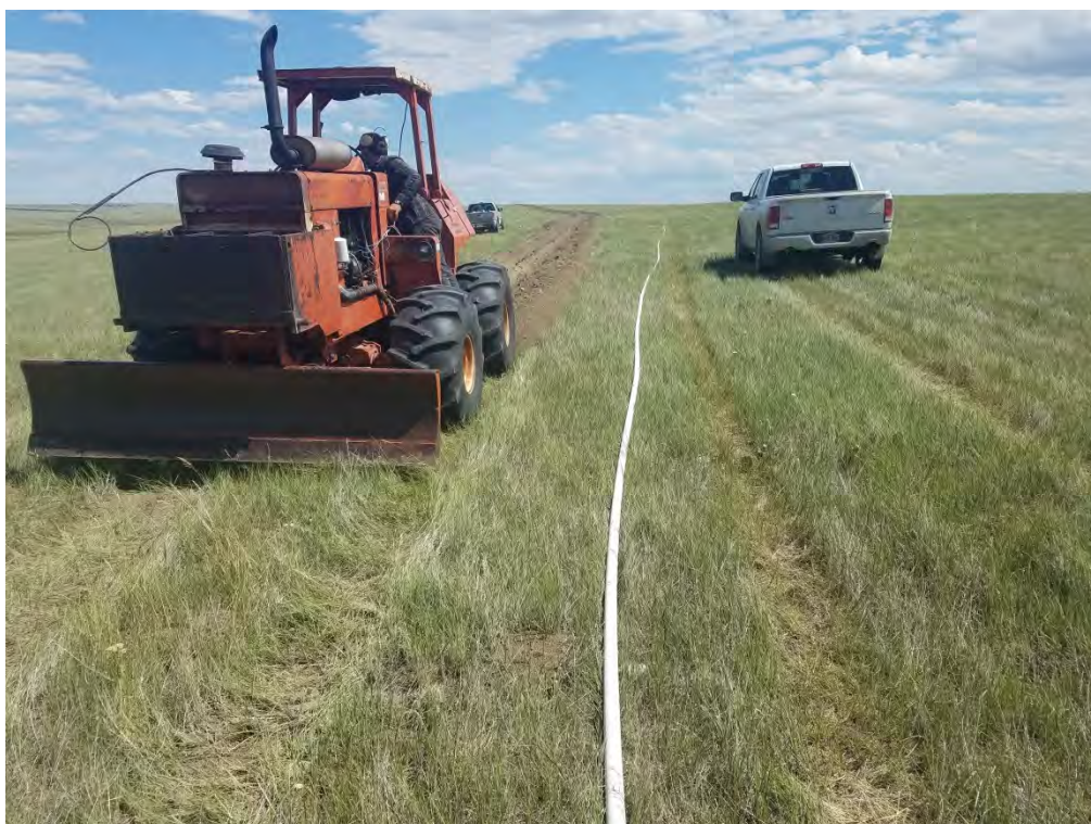
Figure 3-8. Livestock Water Pipeline Installation.
